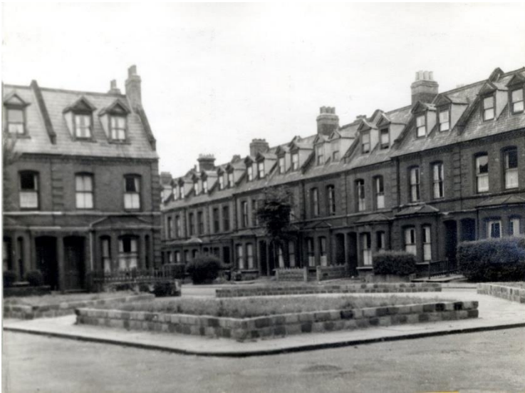
Gilpin Grove and Gilpin Crescent around 1959.
