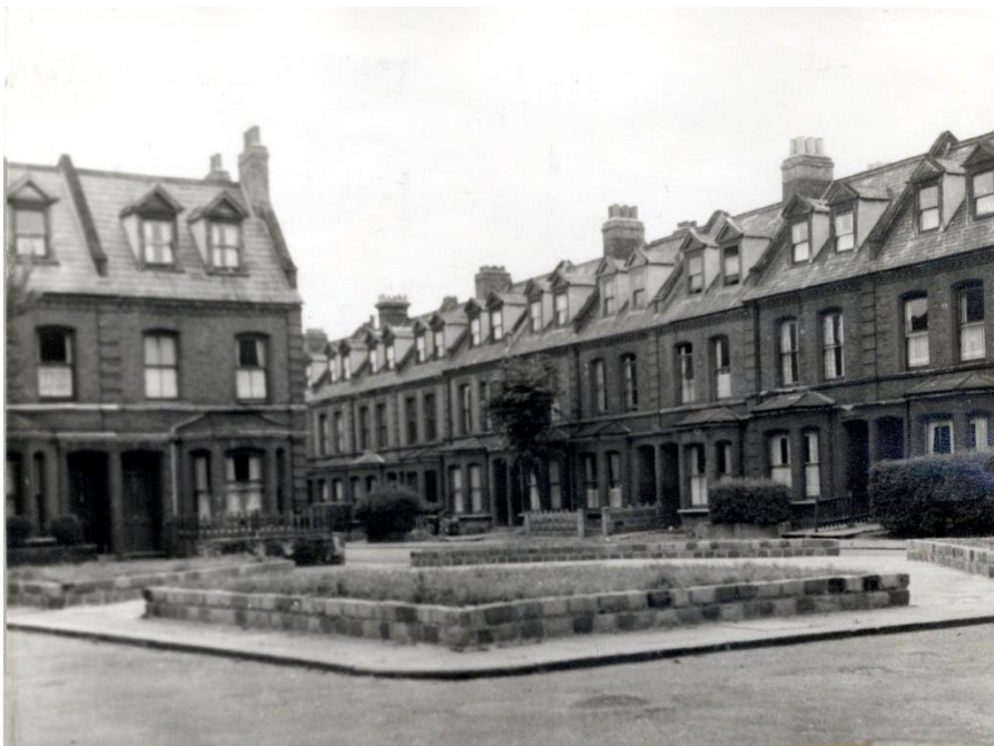
Gilpin Grove and Gilpin Crescent around 1959.
