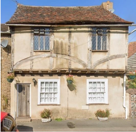
4, Water Lane, Faversham, which was the Elephant and Castle public house
