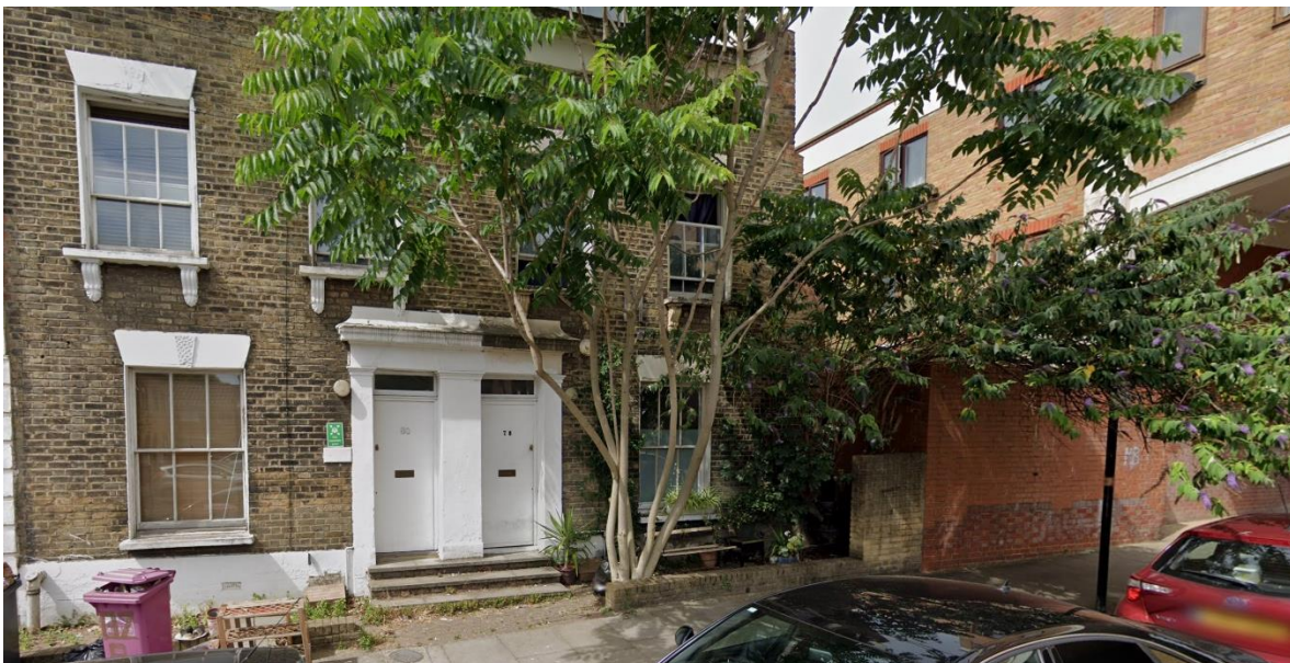
The front of what were 3 and 5 Armagh Road
